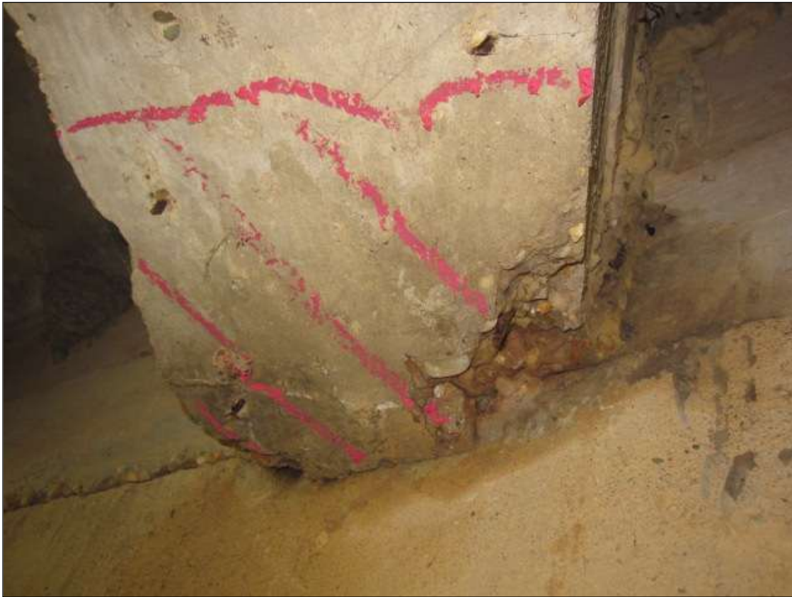
5" X 3" X 1" DEEP SPALL AND 9" X 8" DELAMINATION IN BOTTOM OF BEAM 4 AT ABUTMENT 2
