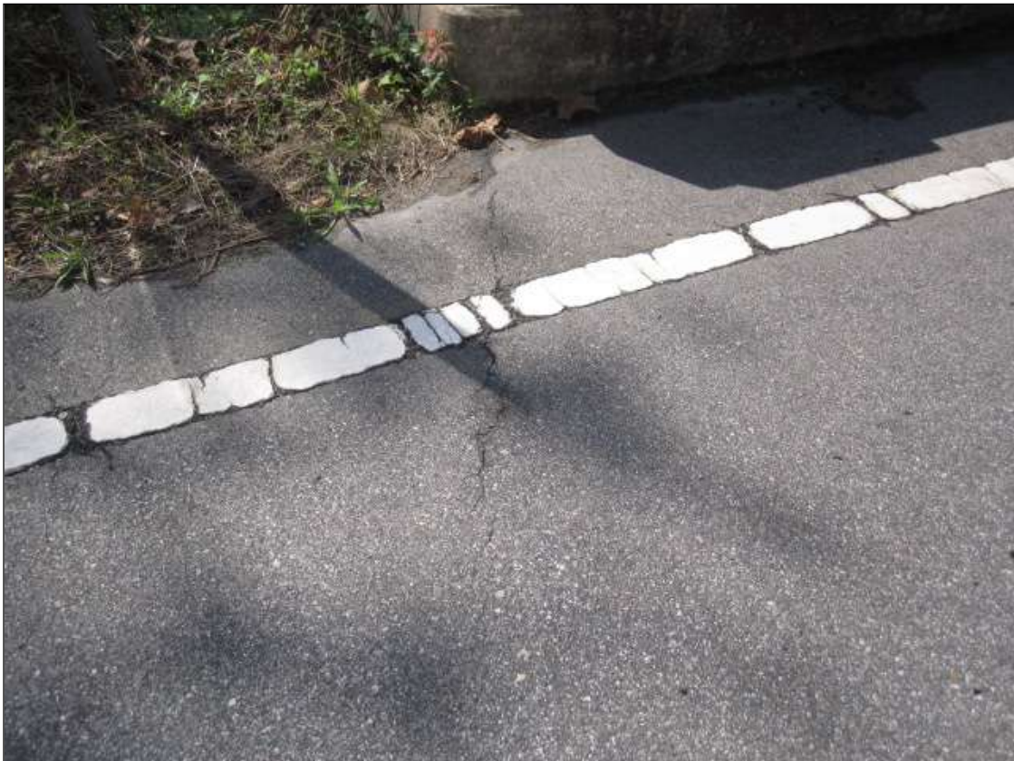
TRANSVERSE CRACK IN ASPHALT WEARING SURFACE ALONG FILL FACE AT ABUTMENT 2
