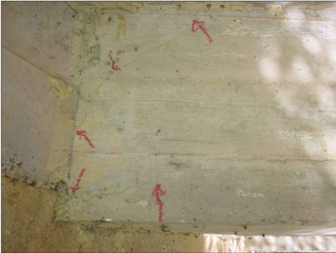
LONGITUDINAL AND DIAGONAL HAIRLINE CRACKS IN SOUTH FACE OF BEAM 7 AT ABUTMENT 1
