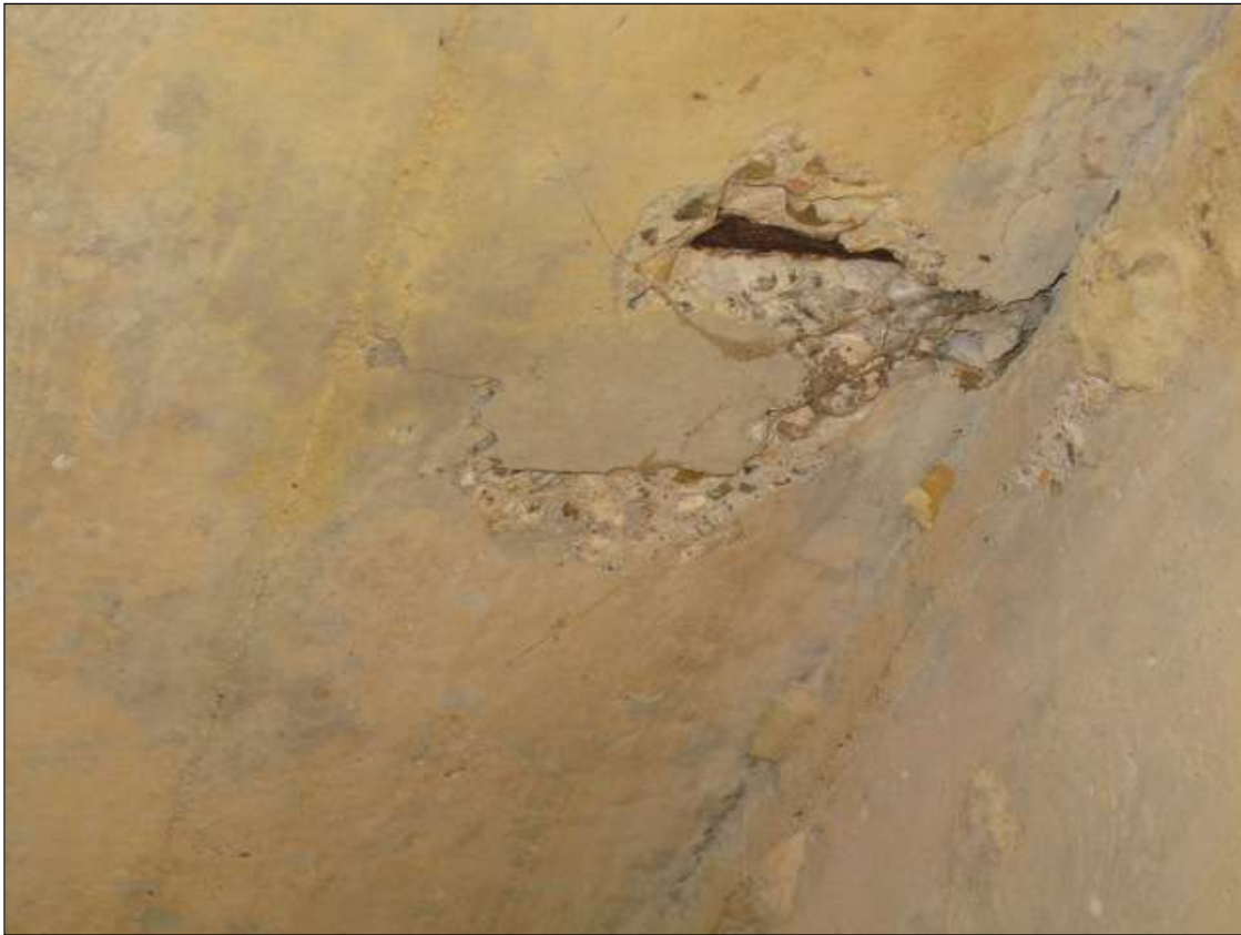
4" DIAMETER X 1/2" DEEP SPALL WITH EXPOSED REBAR IN BOTTOM OF DECK BAY 7 NEAR MIDSPAN
