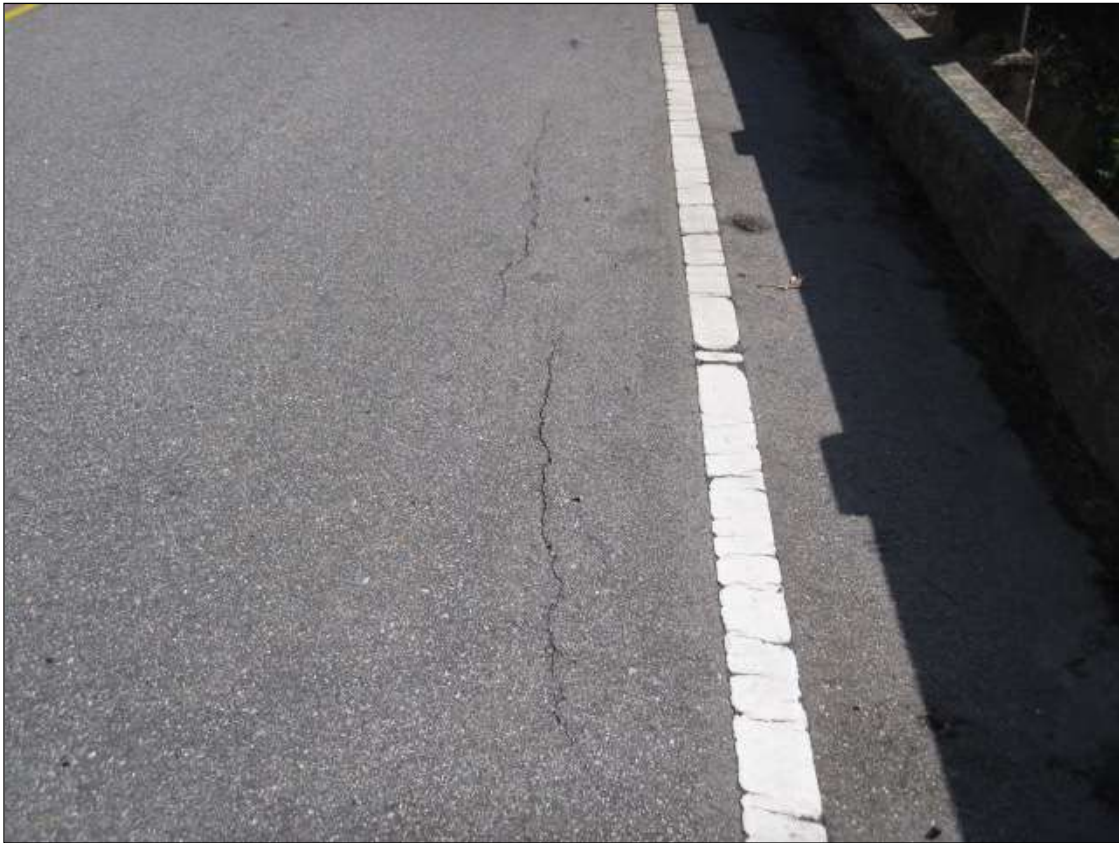
LONGITUDINAL CRACK IN ASPHALT WEARING SURFACE SPAN 1
