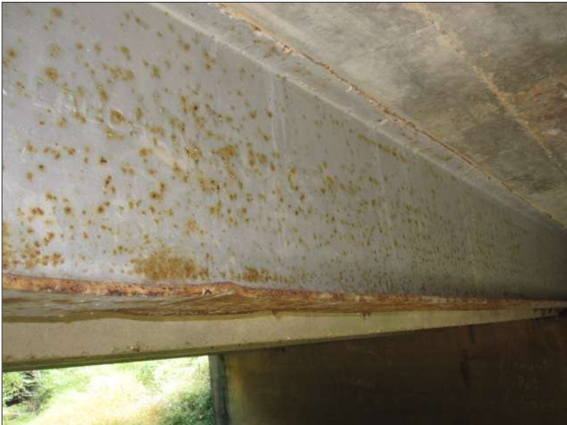
SURFACE RUST ON APPROXIMATELY 15% OF BEAMS SURFACE AREA, BEAM 9 SHOWN
