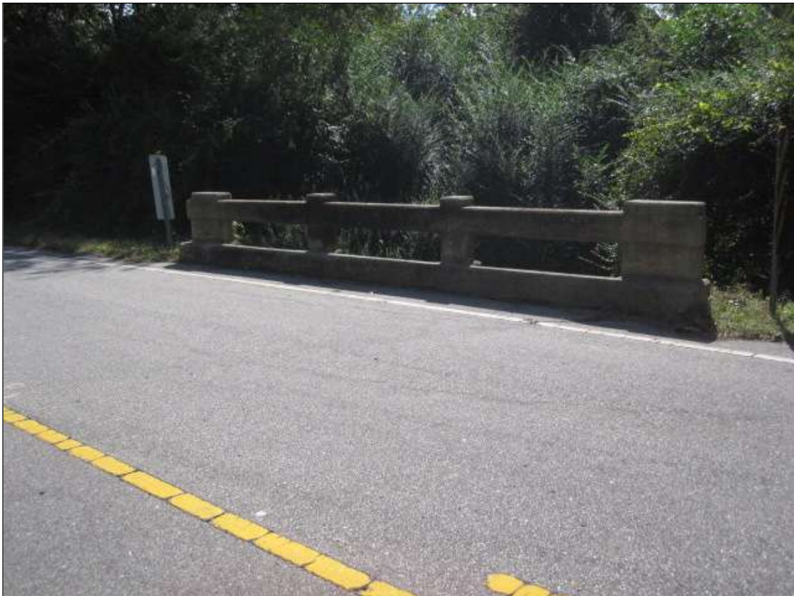
SOUTH BRIDGE RAIL, NORTH BRIDGE RAIL SIMILAR
