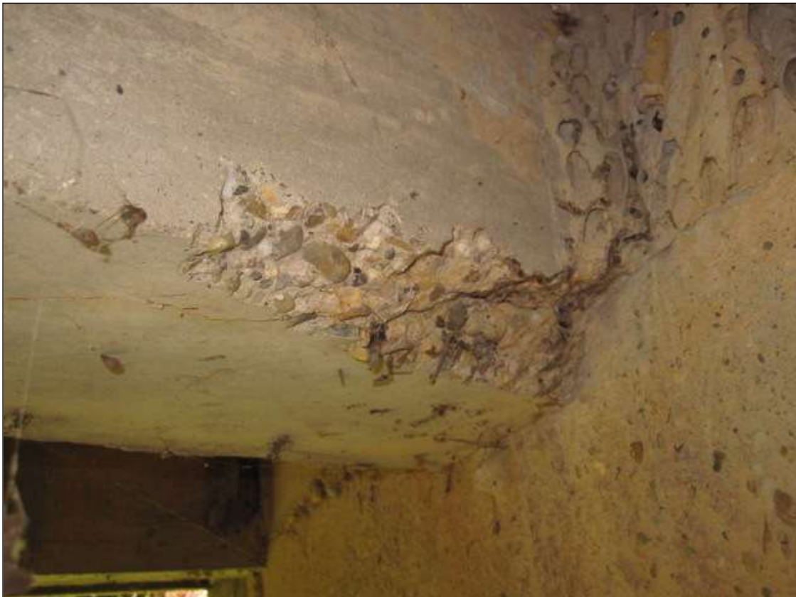
9" X 3" X 2" DEEP SPALL IN BOTTOM OF BEAM 7 AT ABUTMENT 1
